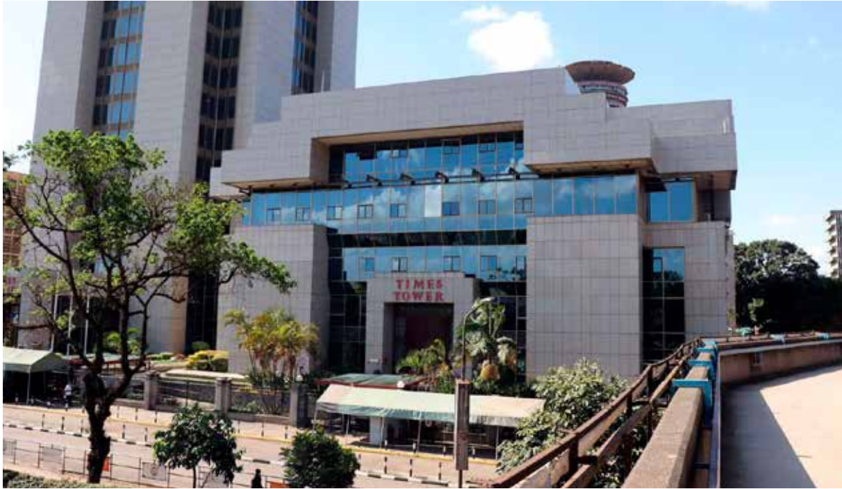
Kenya Revenue Authority building
